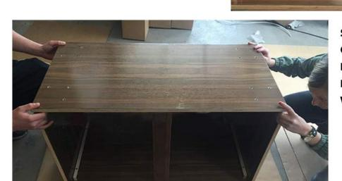
STEP 9: FLIP OVER AND SECURE ON TO SIDES AND BACK, LINING UP GROOVE WITH THE BACK SIDE AND THE DIVIDER WITH THE FRONT DOWEL.
