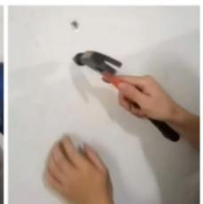
Fix the Mounting Bracket(C) to the hook-shaped expansion anchors with self-tapping screws.
