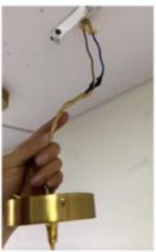
Note: You can either cut off the excess light cord or coil it inside the Ceiling Canopy(E). After connecting the wires, secure them with adhesive tape.
