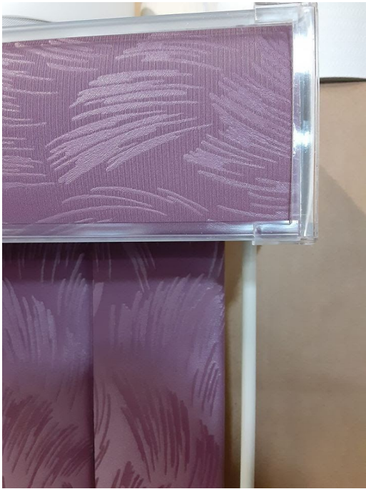
Picture D – valance corner
