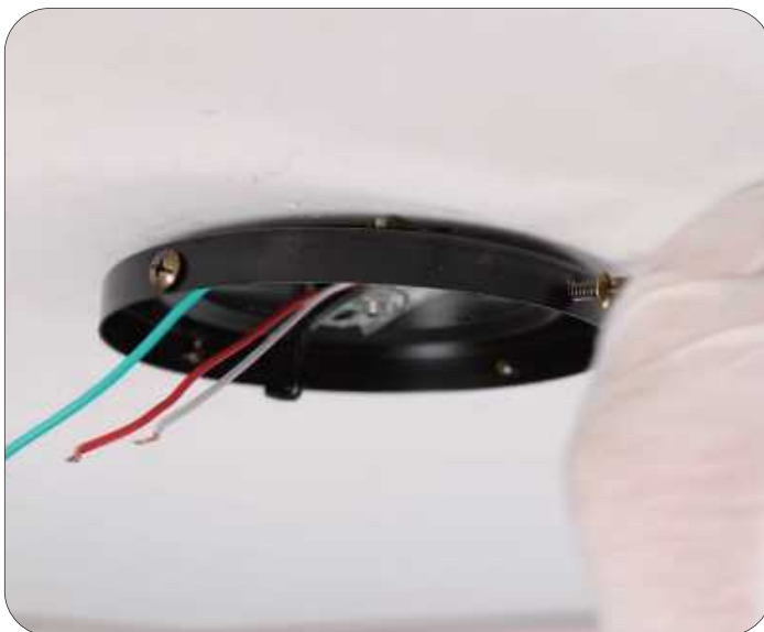
11. Loosen the screws
