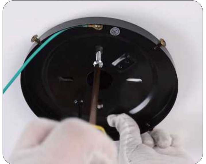
10. Tighten the screws to secure the hanger
