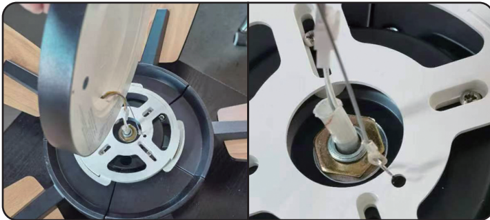
Step 10. Lock the safety rope and connect the wires of the light. (NOTE: The safety rope needs to be locked to the inner ring of the fixture mounting disk)
