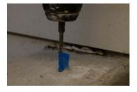
3. Make sure that the holes you have drilled are free of any concrete debris. OPTIONAL: Deposit a small amount of clear silicone into each drilled hole.
