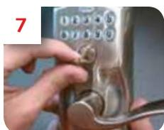
**7** Insert original key and rotate key to the two o'clock position.
