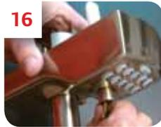
**16** Push cylinder back into keypad lock housing using the follower bar. **Remove the key.**
