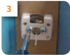
3 Remove deadbolt from packaging using a Phillips screwdriver.
