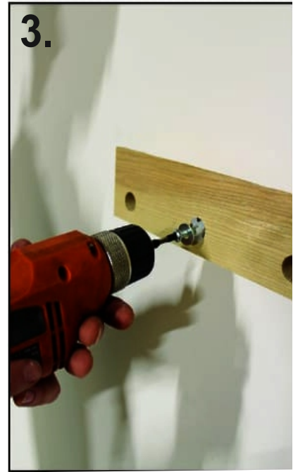
3. Secure the screws tight into the hole drilled in the wall with the help of drill
