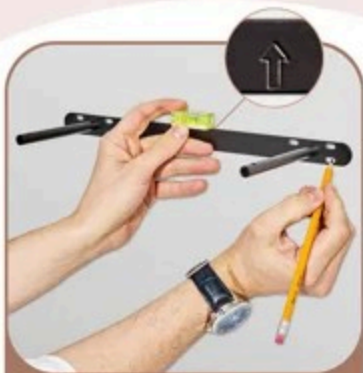
Level Bracket and Mark
