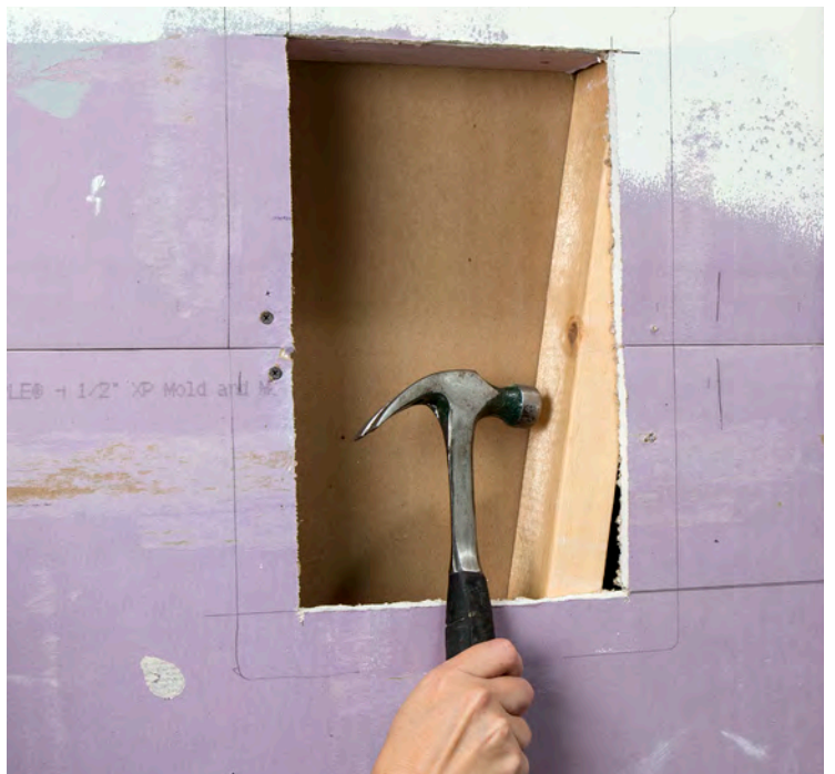
Construct a framed box between the wall studs.
