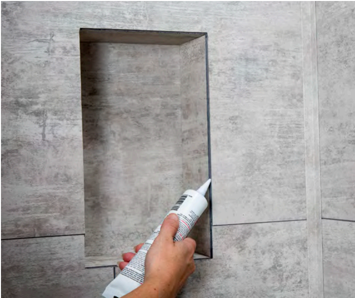
Seal joints with silicone sealant, ensuring a waterproof seal.
