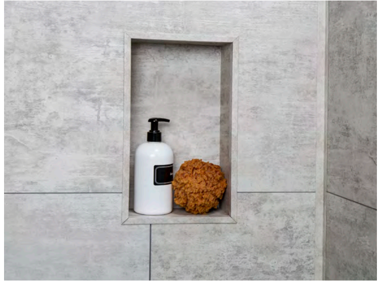
Apply Paliade tiles over membrane lip. Continue applying tiles to complete project. Apply sealant to edges, corners and anywhere else water could penetrate.
