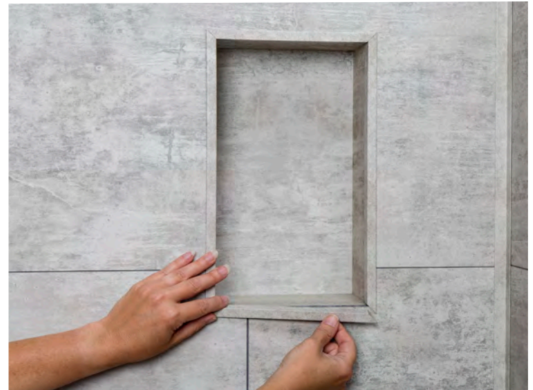
Cut and miter trims to treat the 90-degree connection point of the Paliade tiles. When dried, apply bead of sealant at the inside corners of the niche.
