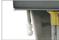
03. Tighten the screws and pipe connector
