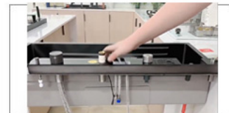
02. Insert the faucet into the sink
