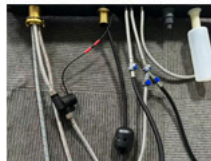
06. Connect the motor with the faucet and fix the position of gravity ball
