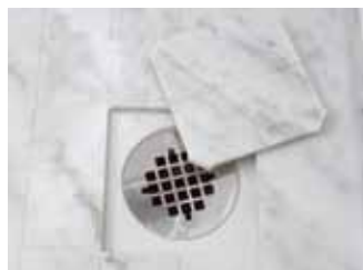
Hidden drain in base
