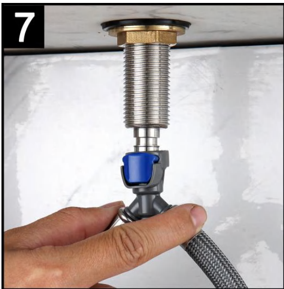
7. Connect the quick connector to the faucet body
