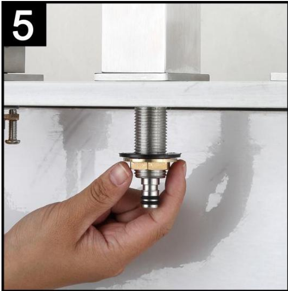
5. Screw the nut and washer to the faucet by your hand
