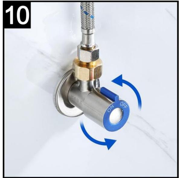
10. Turn on the angle valve and faucet to check if there is any leakage in all the connection parts
