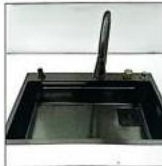
9: Apply sealant around the countertop opening, install the sink where the paste has been injected, place and cover the glue, and place the sink evenly
