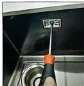
8: Use a power screwdriver to fasten wicker screws to the edges to reinforce the drain.
