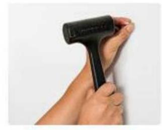
Hammer the expansion screws into the drilled holes.
