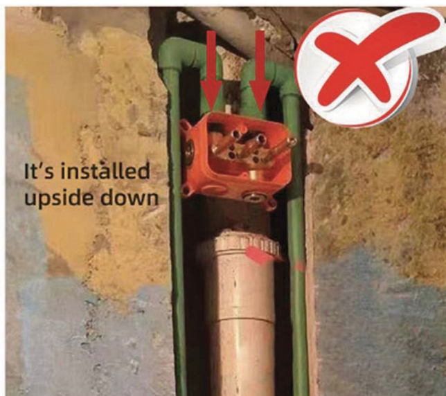
The installation of concealed plastic box in wrong way
