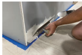
Apply trowel-on adhesive to the wall using a trowel, referencing adhesive directions.
