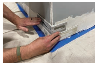
If you are using outside corner pieces, start with them on left side of overall install.
