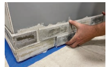
Fit the first piece up to the outside corner piece as tight as possible.
