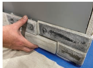
Reaching the right end, with the opposite outside corner in place, you will need to trim the final piece to fit. Note that outside corner pieces have grout seams on both edges. This allows a cut brick to butt into place.
