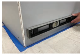
Set a level line above the floor.
