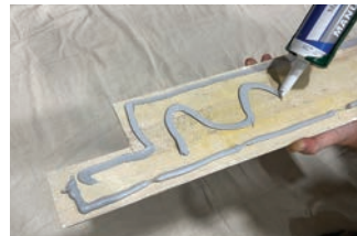
Apply tube adhesive to the back of the panel piece.
