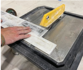
Using a tile wet saw for general cuts.
