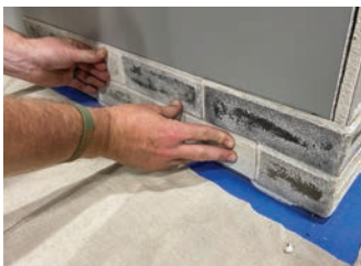
Install the last piece in the first row once it is trimmed to size.
