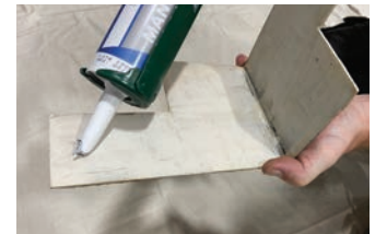
If using tube adhesive, apply to the back of the outside corner piece.
