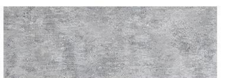
Concrete wall surface
