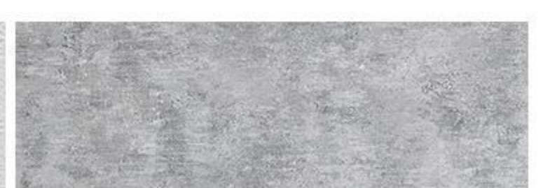
Concrete wall surface
