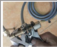
Install gas pipe.
