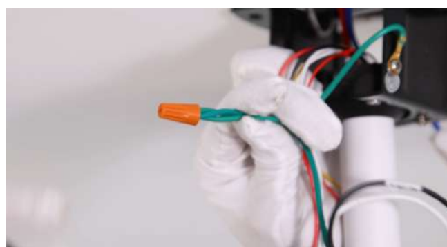
30. Use wire connecting nuts to connect the three ground wires (Green) coming from the downrod, receiver and hanging bracket
