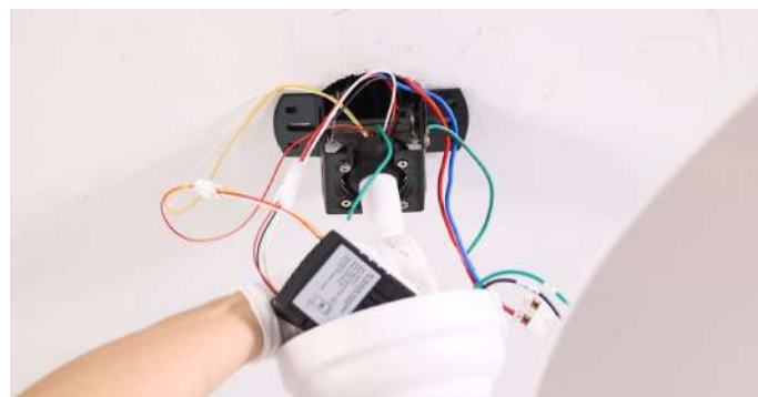
29. Place the downrod ball into the slot in the ceiling bracket. If the slot doesn't align properly then rotate the ball
