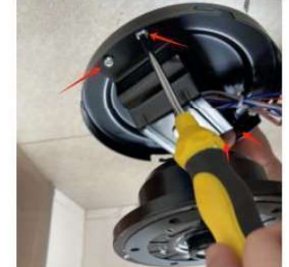
Hang the motor to the ceiling bracket
