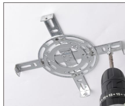
3. Secure each arm of the hanger by fixing them to the ceiling with the help of the wood screws.
