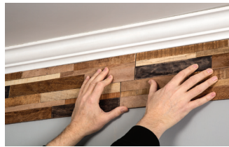
Moving left to right, fitting into the notches of panels.
