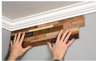
Beginning from inside corner on left, place the first panel.
