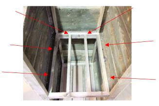
6. Now sit your **roof** on top of your unit and screw together where shown in diagram below.
