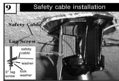
For Canadian installation and for USA fan and light kit combinations over 35 lbs, in both flush and downrod mode the safety cable must be installed into the house structure beams using the 3" lag screws, washers, and lock washers. provided. Make sure that when the safety cable is fully extended the leadwires are longer than the cable and no stress is placed on the leadwires.
