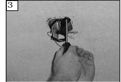
Use metal outlet box suitable for fan support (must support 35 lbs). Before attaching fan to outlet box, ensure the outlet box is securley fastened by at least two points to a structural ceiling member (a loose box will cause the fan to wabble). Use only the screws provided with the outlet box.
