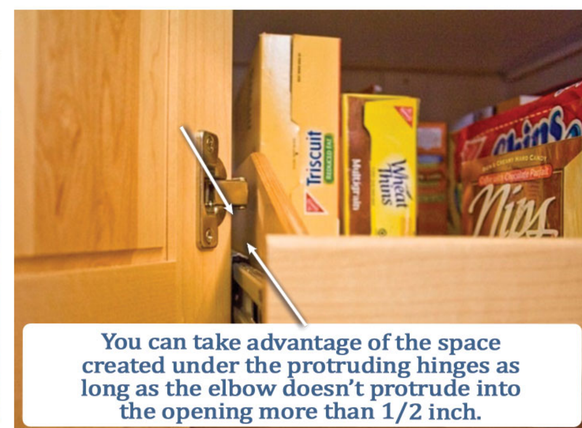
Must be 1/2" or less to be able to ignore the hinge elbow and measure from the door edge.
