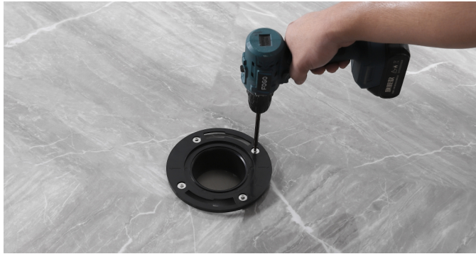
5. Place the fixed disk into the drain outlet and tighten the screws to secure it.
