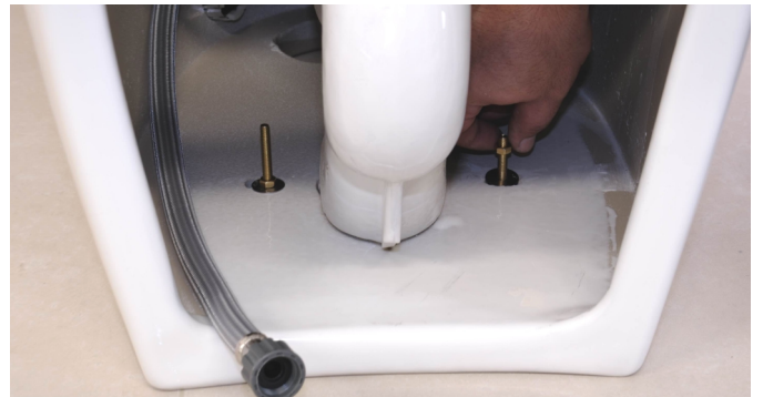
14. Make sure two holes in the bottom of the toilet align with the two long screws in the fixed disk, then install it.
