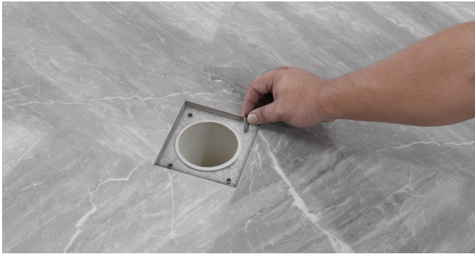
4. Put the screws into the holes.
