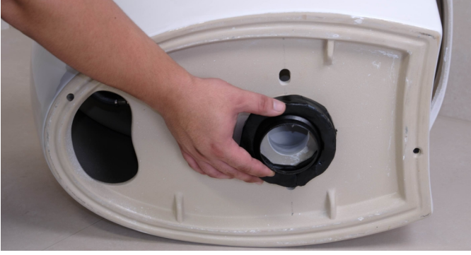
11. Gently turn the toilet over to access the base and install the flange ring.
