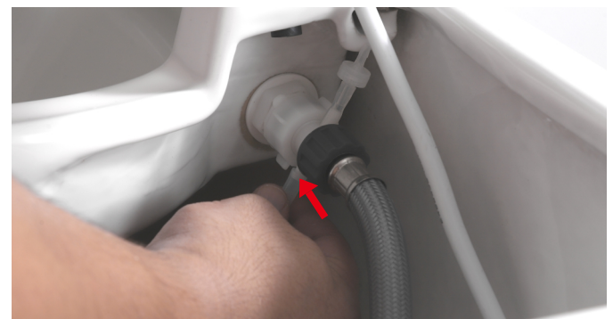
15. Put the toilet lid in the toilet, reconnect the hose, the transparent pipe and the black wire.
