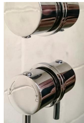
9. Re-fit the Temperature Handle Concealing cap.
