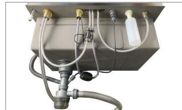
Waterfall Sink installation finish!!!
