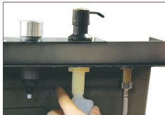
02.Installation of fixed soap dispenser
