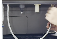
03. Connect the cup washer with the hose
