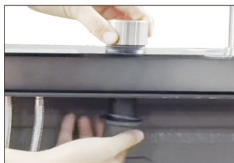
02.Install in the sink by tightening the screws on top and bottom
