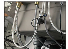
06. Connect the motor with the faucet and fix the position of gravity ball
