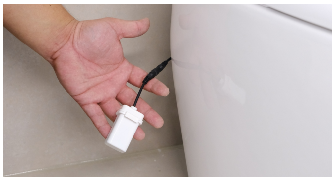
Step 3. Connect the 9V spare battery to the toilet's connection cable and place the battery in a dry area behind the toilet.
