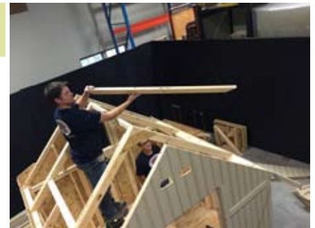
Install rear rafter where marked using 2 1/2" screws.
