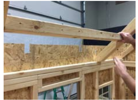
Locate and fasten double 2x3 T-bar where marked on trusses, with 2 1/2" screws.
