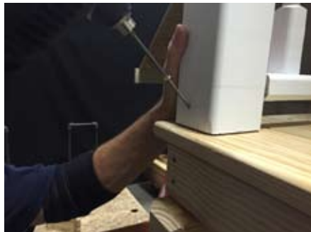
Fasten railing post to deck with 2 1/2" screws.
