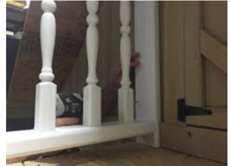
Back against the building 1" in from side of deck.
