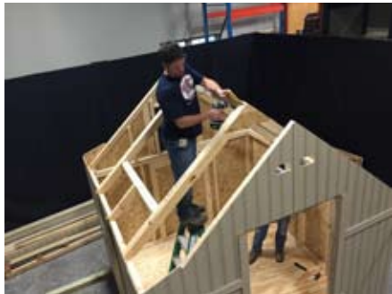
Fasten short rafter on front wall and double T-bar. Fasten ridge T-bar using 2 1/2" screws.
