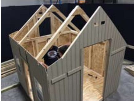
Trusses are in place.
