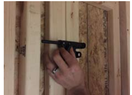
Install latch on inside of door with black screws.
