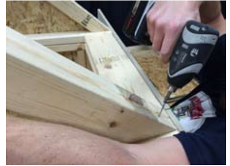
Back wall. Fasten using (3) 2 1/2" screws.
