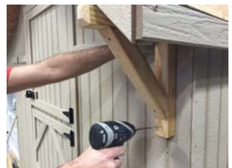
(2) brackets against corner trim up against the rake.
