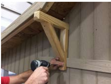
Fasten brackets with 2 1/2" deck screws, install in pocket of the trim, square it and push it up against the rake.
