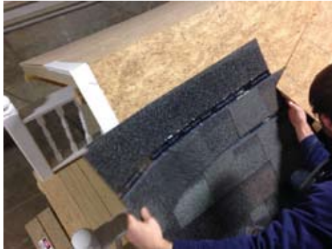
Shingle underneath dormer.
