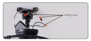
White(neutral) supply wire to the white wire Black (live) supply wire to the black wire Green supply wire to the green wire Then use the wiring cups to cover the wiring connection points
