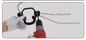
For Concrete Ceiling, first use 8mm drilling bit to drill hole according to the length of the expansion screw, then fix the handing bracket with the expansion screw on the ceiling.
