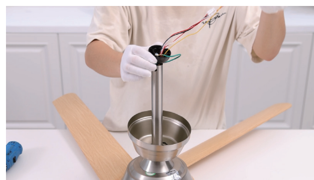
21. Put the hanger ball through the downrod
