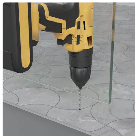
3/ Drill holes at marked locations
