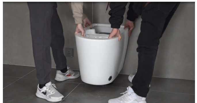
11. Move the toilet to the location where it will be installed
