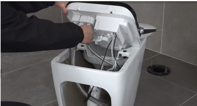
8. Take off the whole toilet seat and unscrew the flexible tube and black wire
