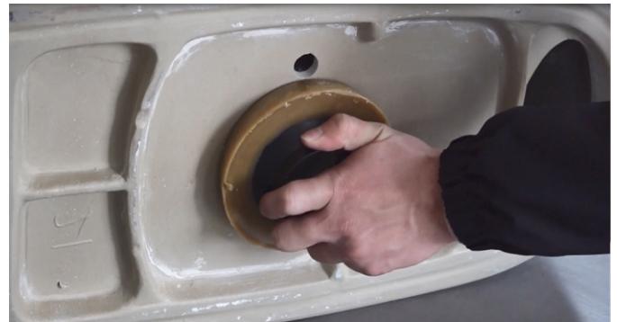
9. Turn over the toilet bowl and install the fixed disk as shown in the figure.
