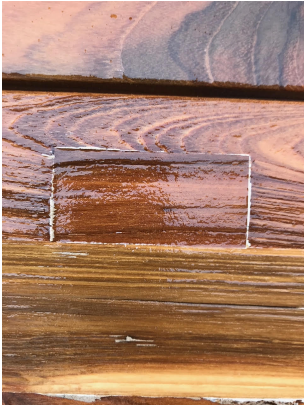
GLUE LINE AT PATCH WHEN INITIALLY WET
