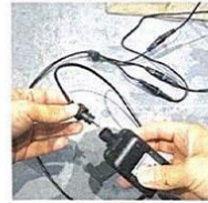
Connect the main wire of the junction box to the transformer.
