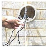
Pull the water pipe out from the circular hole.
