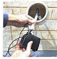
Connect the water pump to the water pipe.
