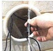
Thread the wire through the hole and pull it out from the circular hole at the back.
