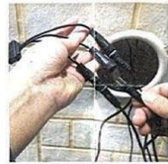
Connect the wires to the junction box.
