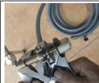
Install gas pipe.
