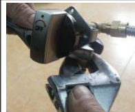
Remove propane pipe
