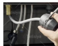
02. Fix the gravity ball at the proper position of the faucet pipe
