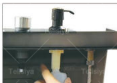
02.Installation of fixed soap dispenser
