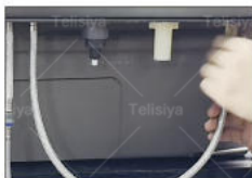
03. Connect the cup washer with the hose
