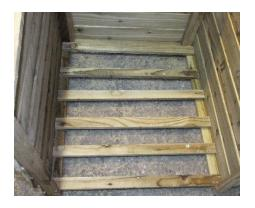
4. Using the spacer as shown in below diagram, screw baton into place using 4 screws provided. Insure the spacer (marked X) is inserted under the lip please see below diagram.
