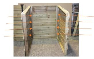
3. Place the 6 floor batons evenly spaced from front to back (please ensure front and back batons are as far forward and back as possible) as shown in the picture.
