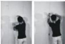
1. Based on the center position between hot water outlet and cold water outlet on the wall and the installation height, place the shower onto the wall to determine the position of hook. Use a marker to mark the position of the hook.
