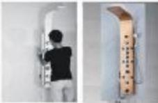
3. Fix the accompanied elbows onto the hot water outlet and the cold water outlet, and then connect the hot and cold water pipes on the back of the shower with the elbows and tighten them using a tool or your hand.
