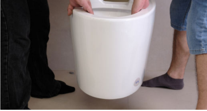
11. Move the toilet to the location where it will be installed.
