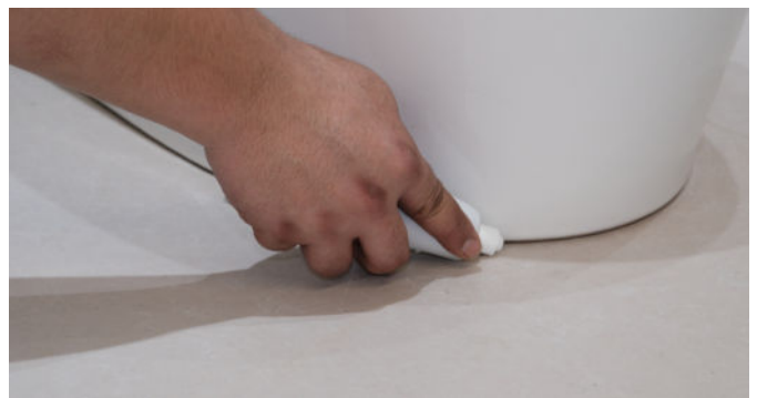
15. Apply some silicone sealant to fix the toilet and insulate the outside dirt from entering. ( The silicone sealant adhesive in the picture needs to be purchased by oneself. )
