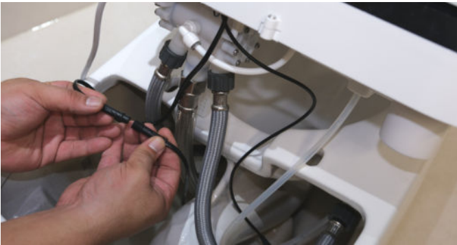
13. Put the toilet seat in the toilet and reconnecting the flexible tube and the black wire.
