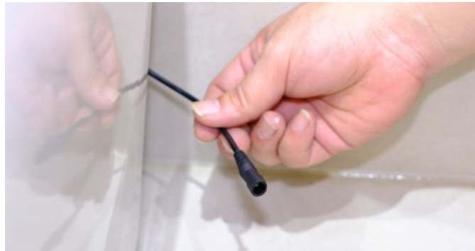
Step 2. Cut off the power supply and find the power outage flushing wire interface behind the toilet.
