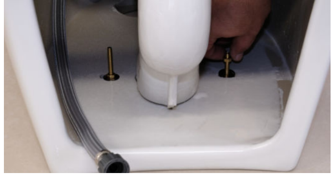
12. Make sure two holes in the bottom of the toilet align with the two long screws in the fixed disk, then install it.
