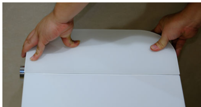
Step 5: After putting the foam bottle into the empty slot, reinstall the back cover of the toilet in its original position.
