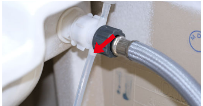
13. Put the toilet seat in the toilet and reconnecting the flexible tube and the black wire.
