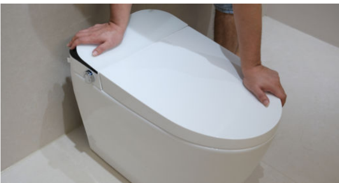
14. Press the lid slightly harder to fix it on the ceramic.
