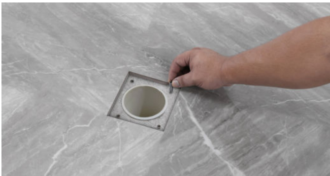
4. Put the screws into the holes.
