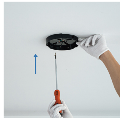
4.Tighten the motor cover to the ceiling with screws
