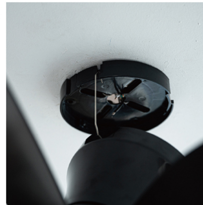
6.One end of the safety hook is linked to the motor one end is connected to the motor cover
