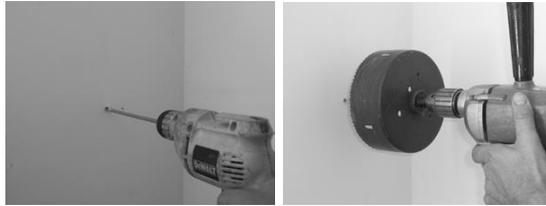
Outside the building, find the pilot hole. Using a hole-saw, with the pilot hole as a guide, drill a 6 1/4” hole.
