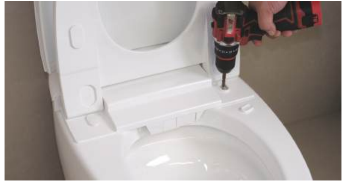
17. Reinstall and fix the positioning screws and the decorative cover.
