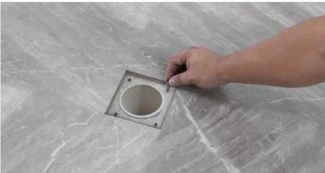
4. Put the screws into the holes.
