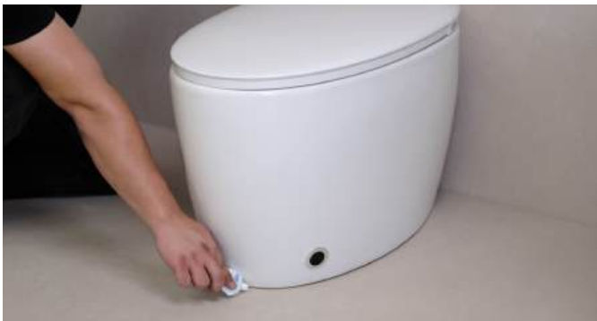
18. Apply some silicone sealant to fix the toilet and insulate the outside dirt from entering. ( The silicone sealant adhesive in the picture needs to be purchased by oneself. )
