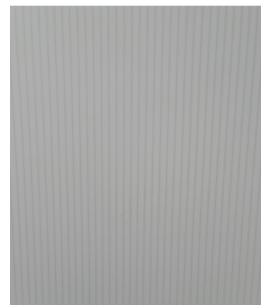
photo of the 4mm roof panel
