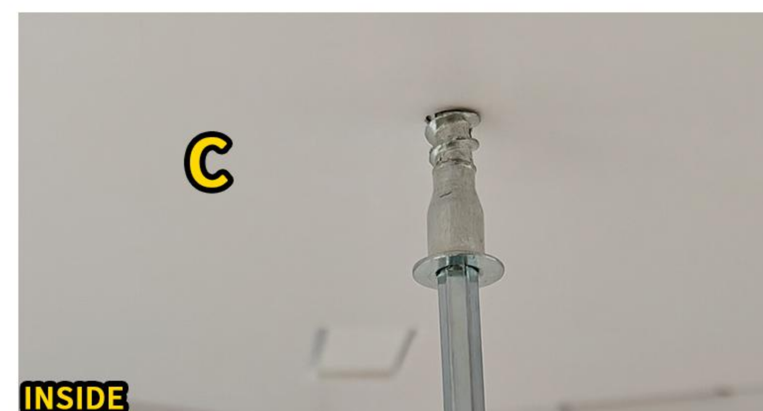
12. SCREW IN 3 SCREWS AT THE JOINT BETWEEN BOARD B AND BOARD C
