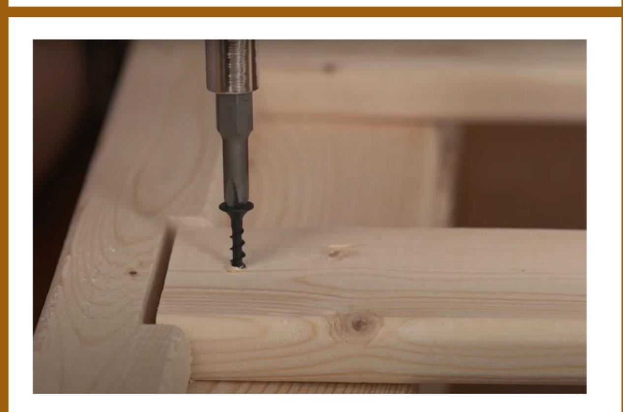
7. Secure the cross supports using the 1 1/4" screws.
