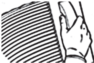
Figure 6 - Using a notched trowel. Angle the trowel at a 45 degree angle to ensure that a full ridge is made with the notches.
