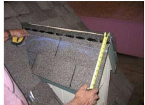
Once the last row is installed measure 4 1/4" from the top down and snap a chalk line. This ensures a straight line for the cap.
