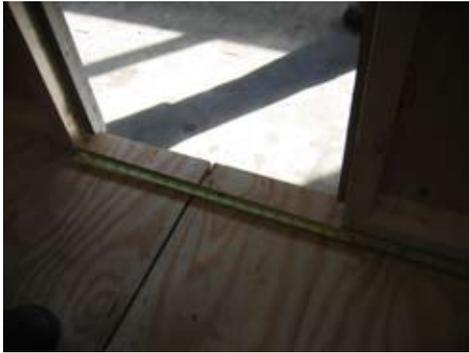
Be sure to measure from 2x3 to 2x3 that the opening is 20". Do not measure in between the door stop. If it is not you may need to adjust it one way or the other.
