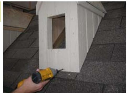
Fasten the dormer onto the base.
