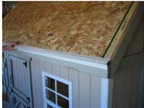
Install drip edge all around the edge of building as shown.
