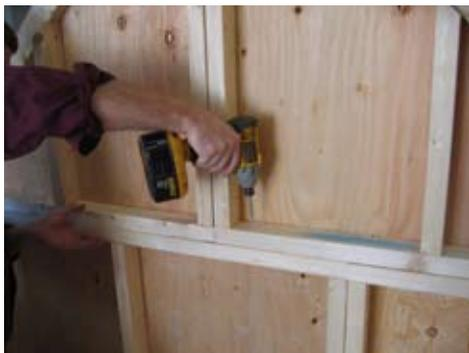
While someone presses in on the outside fasten on the inside. Put 2 1/2" screws on either side of the splices to provide strength.
