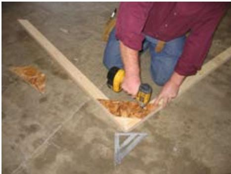
Fasten the truss gussets, keep the top even. Use black headed screws for this. Install one gusset on either side of the truss. For a total of 2 per truss.
