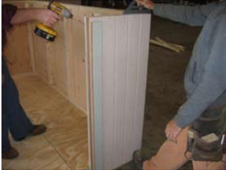
Install panel K. Measure in between these two panels. From 2x3 to 2x3 it should measure 34".
