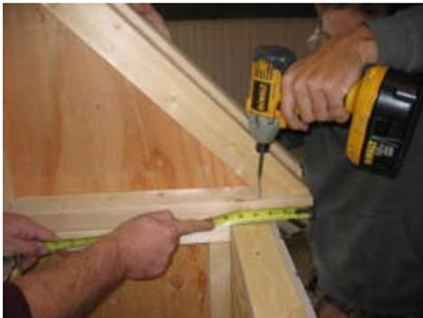
Measure in 5 1/2" from the outside as shown. Be sure to pull in against siding and fasten as shown.
