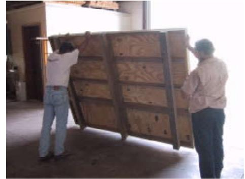
Turn the floor on the back with the plywood facing up. Make certain that the ground is level where the floor sets or you may have problems with the panels or the roof.
