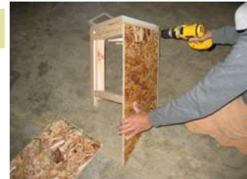
Fasten one side of OSB to trusses.
