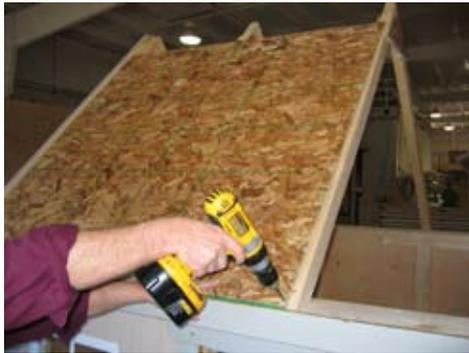
Install first sheet of OSB (orient strand board) sheathing. Fasten only on the bottom first. Refer to layout diagram for your specific building. Use black-headed screws to fasten.
