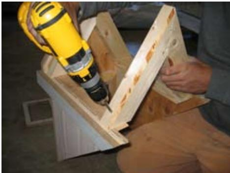
Fasten small truss as shown.
