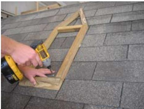
Screw the base into the roof. You can use 2 1/2" screws. Be sure to check on the inside and break off the screw that is exposed.
