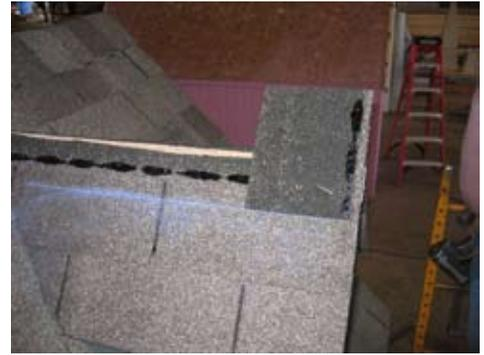
Start by installing a starter cap.
