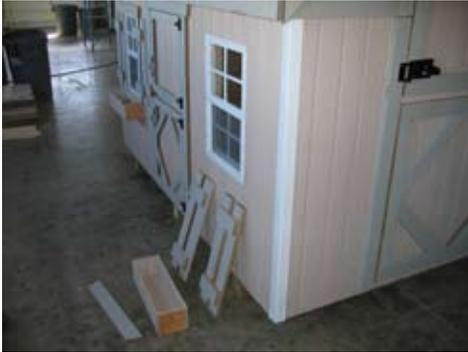
Install the corner trim with small white nails. Be careful to not “wrinkle the corners” when installing.
