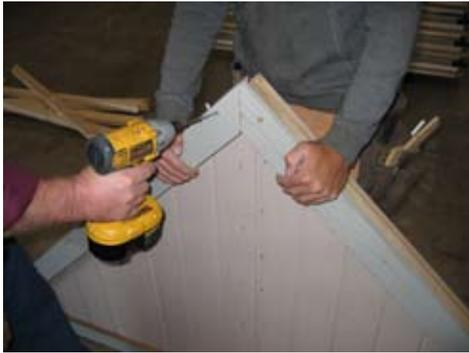
Press together trim as shown and fasten. The trim is not fastened to allow for adjustments.
