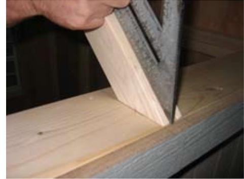
Truss should fit as shown. Make sure truss does not go past the edge of the 2x6 onto the trim.
