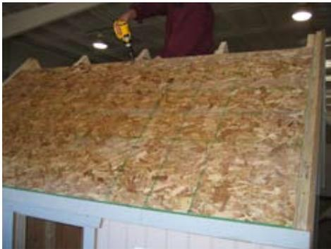
Note gap between OSB and 2x2 with trim. Be sure you have this before fastening on top.
