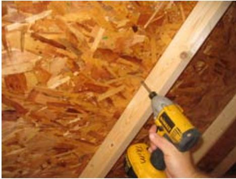
Once the frame is fastened on the outside you can break screws poking through the roof. You can also fasten the frame from the inside out.
