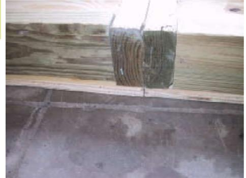
Make sure the plywood is even before fastening. If it is not, you will have an uneven floor.
