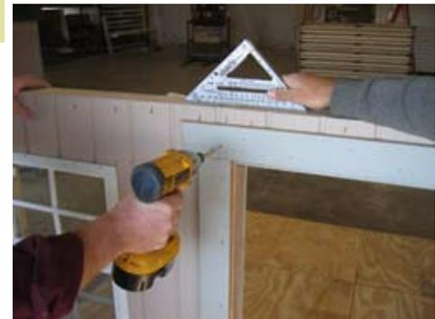
Fasten the other side of the header block B to panel C.
