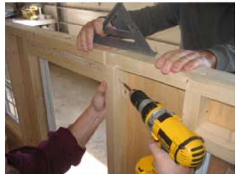
Install panel C. Fasten this onto the header block as shown.
